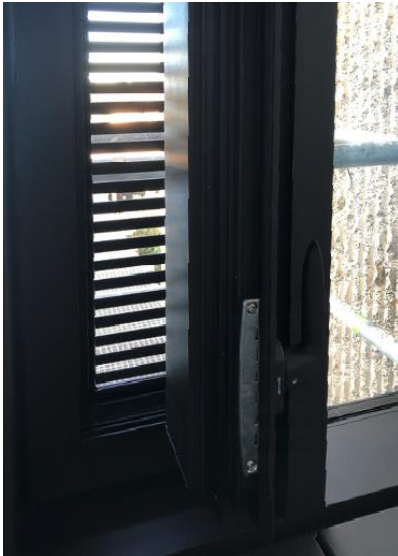
Ventilation naturelle (flap)
